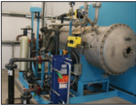
Photo 2 – LOX/GOX Pad Photo 3 – Ozone Generator
