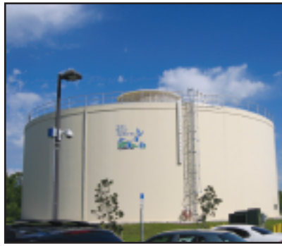
Photo 7 – Ground Storage Tank
