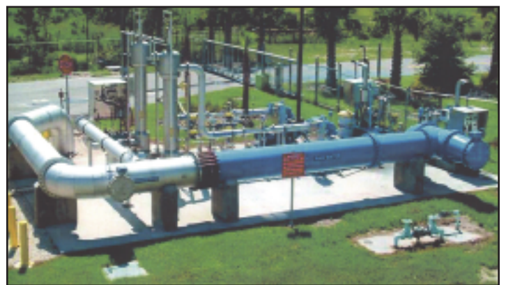
Photo 5 – Ozone Injection Pad
