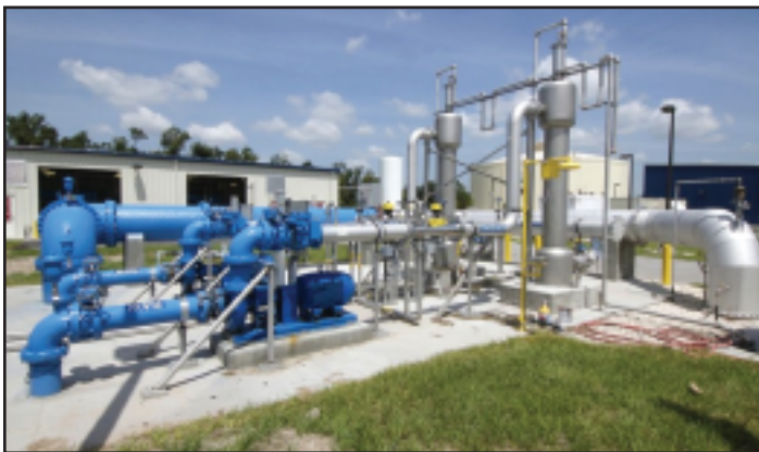
Photo 4 – Ozone Injection Pad
